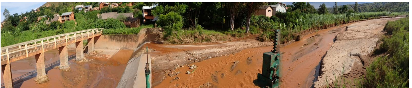
Figure 5. Wier on the Ibizy River in the Ambohimandroso Village, indicating how widespread the siltation of watercourses is in the region
